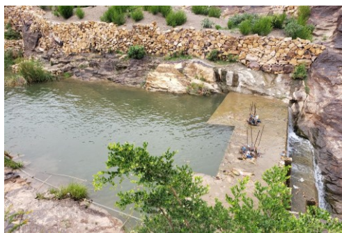
Surface dam in-- Al-Selw district, Taiz | Photo Credit: UNDP
