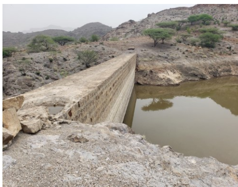
Potential Project Site: Small gravity dam in Al-Mosaymer district, Lahj | Photo Credit: UNDP
